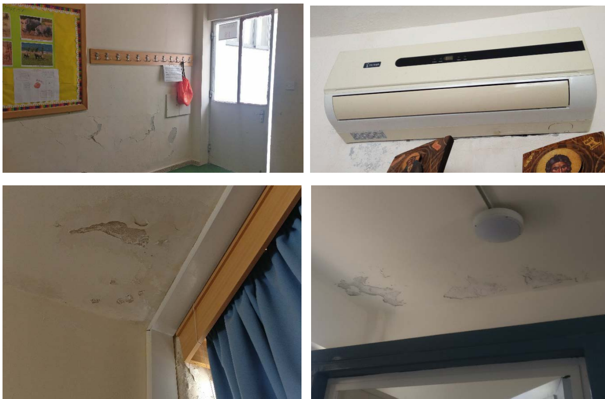
FIGURE 28: CONDENSATION AND HUMIDITY PROBLEMS PRESENTED IN VARIOUS SPACES OF THE PILOT SCHOOLS
