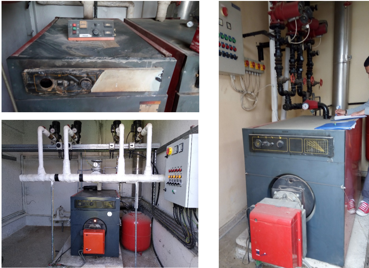
FIGURE 30: INDICATIVE OIL BOILERS LOCATED AT PILOT SCHOOLS. UP LEFT: DESTROYED BOILER AT AYIOS GEORGIOS SCHOOL. DOWN LEFT: LIVADIA [CB] BOILER. RIGHT AYIOS ANDREAS [CA] BOILER.
