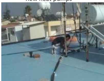
PP2 – Thermal insulation and new solar thermal water heater
