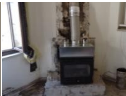
PP7- New efficient fireplace (air module)
