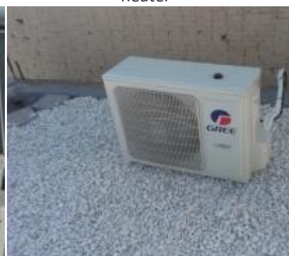
PP12 – New efficient air conditioning compressor
