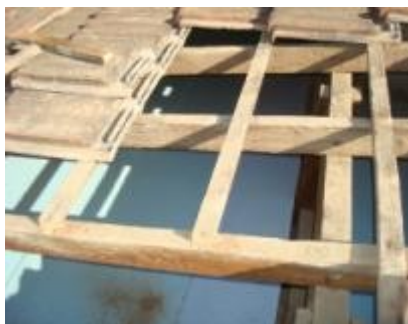
PP16 - Thermal insulation of the roof
