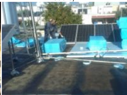
PP9 – Roof thermal insulation and photovoltaics
