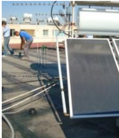
PP4 – Waterproof Insulation and new solar thermal water heater
