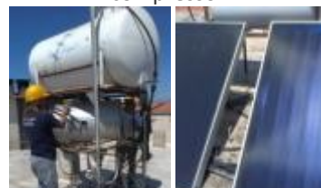
PP14 – Installation of Solar water heater
