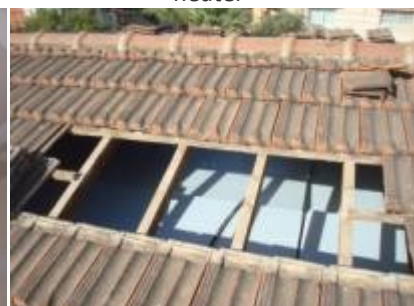
PP16 – Thermal Insulation of the roof
