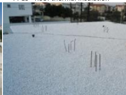
PP20 – Roof with thermal insulation
