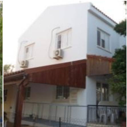
PP25 – After thermal plaster
